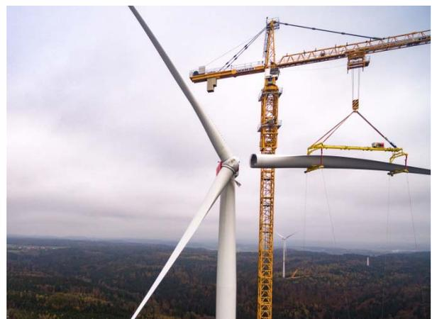
Figure 4: Attaching the leaves. Foto: © Max Bögl Wind AG, photographer: Holger Hessenthaler.
