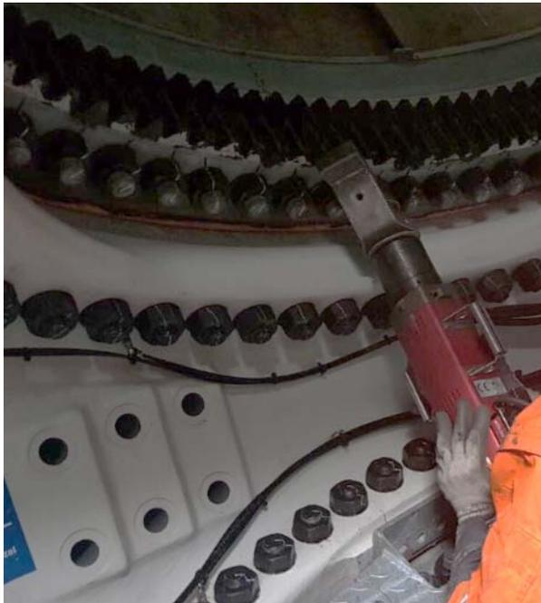
Figure 2: The alkitronic EF 300 Plus in use at the rotor blade bolting.
